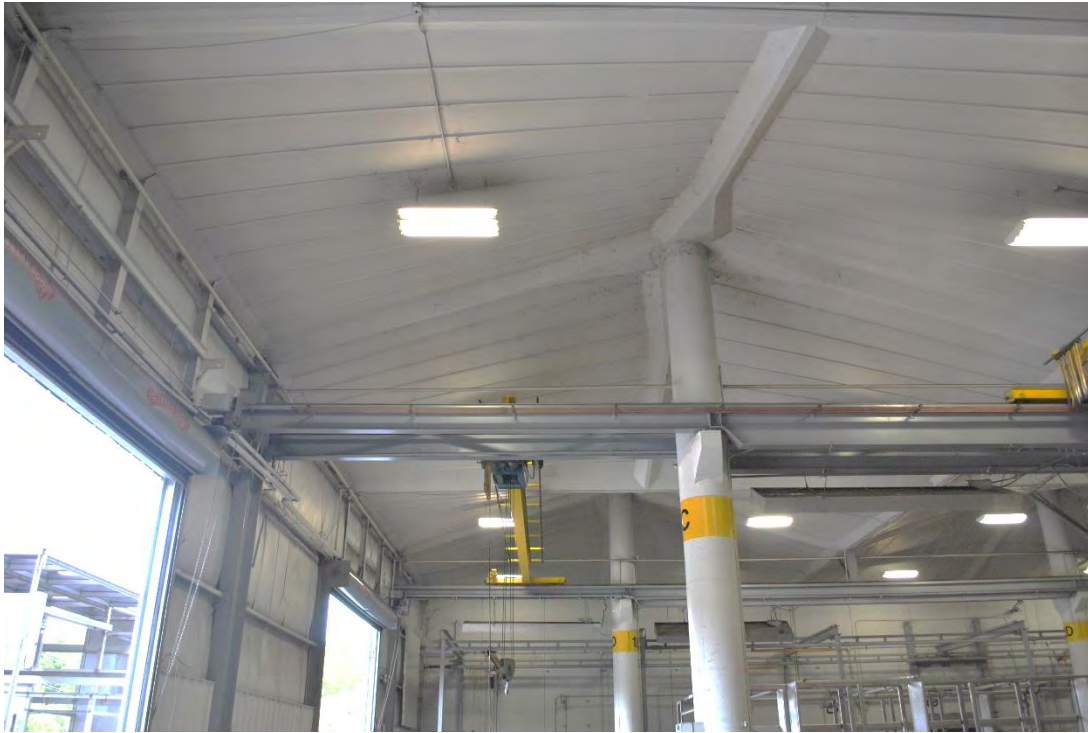
Aeroglide Corporation Building, 1964 Production Room, Ceiling and Structural System.
