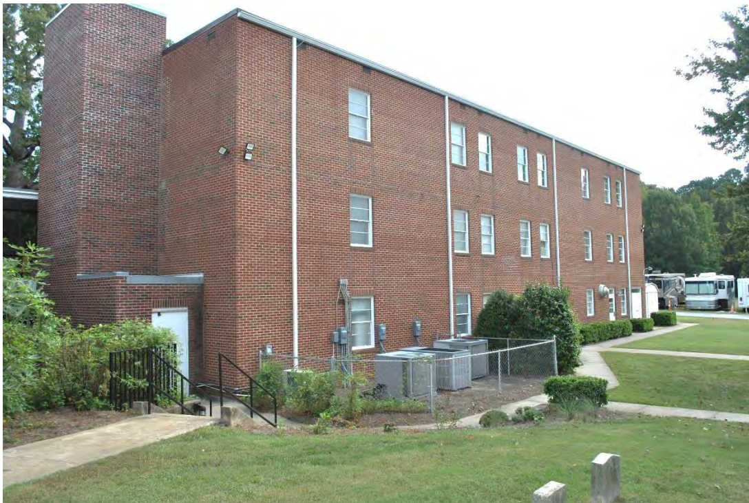
Ephesus Baptist Church, 1964 Education Building, West and North Elevations, Looking South.
