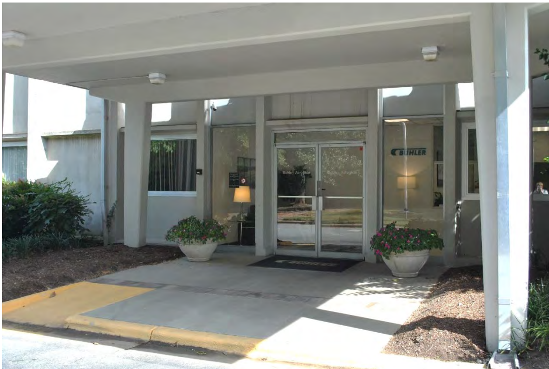
Aeroglide Corporation Building, Main Entrance, Looking East.
