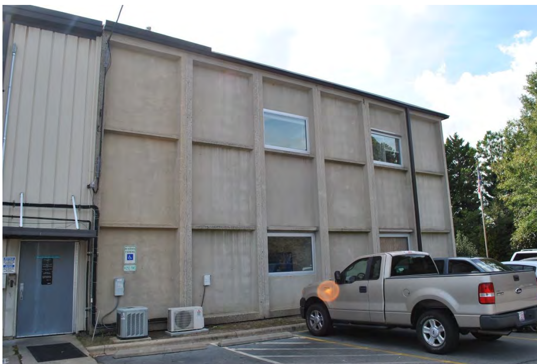
Aeroglide Corporation Building, North Elevation of Office Section, Looking Southwest.
