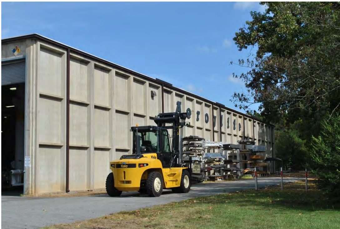
Aeroglidge Corporation Building, South Elevation Showing Original Aeroglidge Sign, Looking Northeast.
