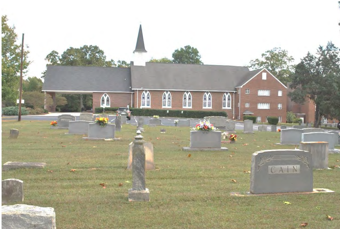
Ephesus Baptist Church, Overall View, West Elevation, Looking East From Main Cemetery.
