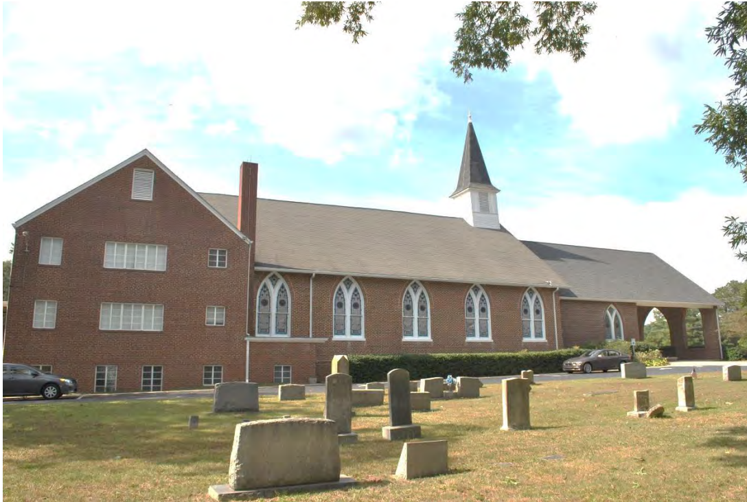
Ephesus Baptist Church, Overall View, East Elevation, Looking West From Cemetery on East Side of Tract.
