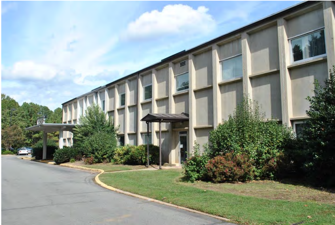
Aeroglide Corporation Building, Façade (West Elevation), Looking Northwest.
