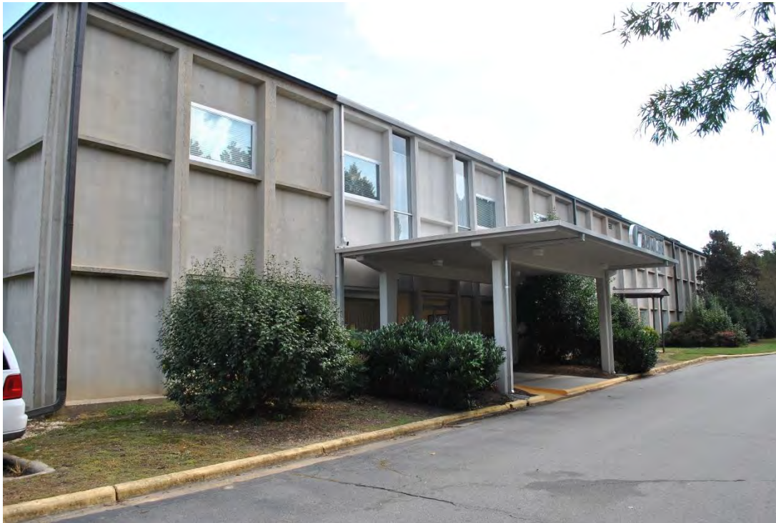
Aeroglidge Corporation Building, Façade (West Elevation), Looking South.
