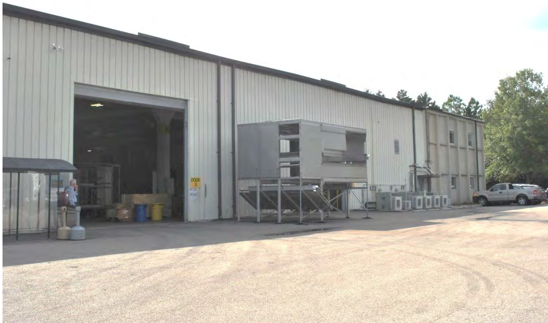
Aeroglide Corporation Building, North Elevation of Production Area (Office Section on Right), Looking Southwest.
