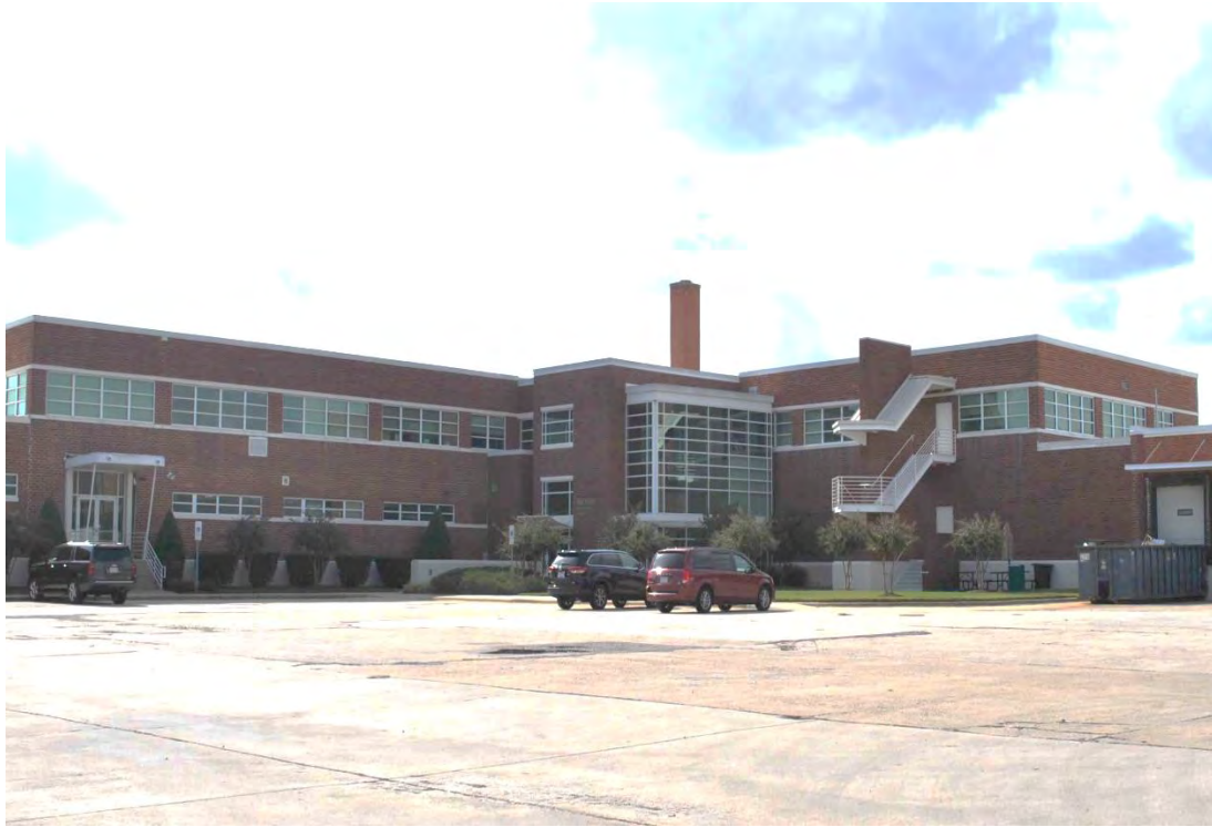
Peden Steel Plant (1956 and 1962), Administrative Wing, Rear and Side Elevations, Looking West.
