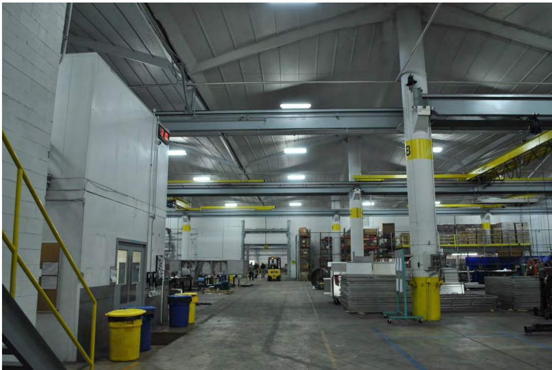
Aeroglide Corporation Building, 1964 Production Room.
